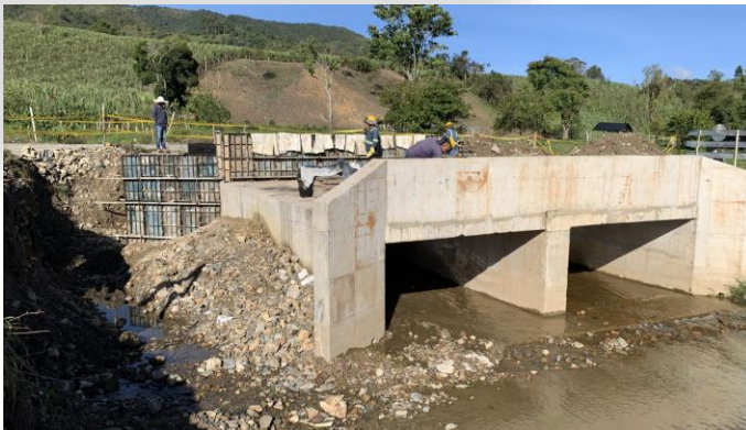
PR37+700. Box culvert doble
