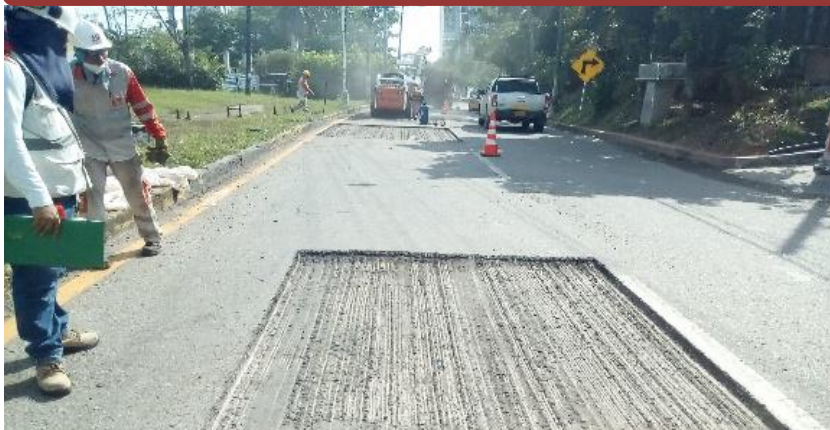
FRESADO DE AS COPAS PR 2+750 AL PR 1+257,8
